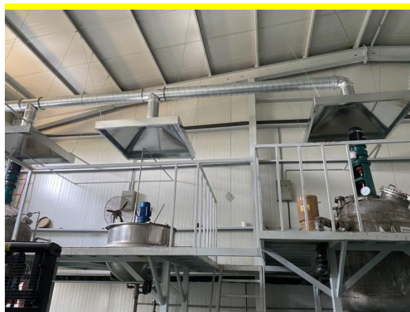
酶解、蒸煮工序集气罩
